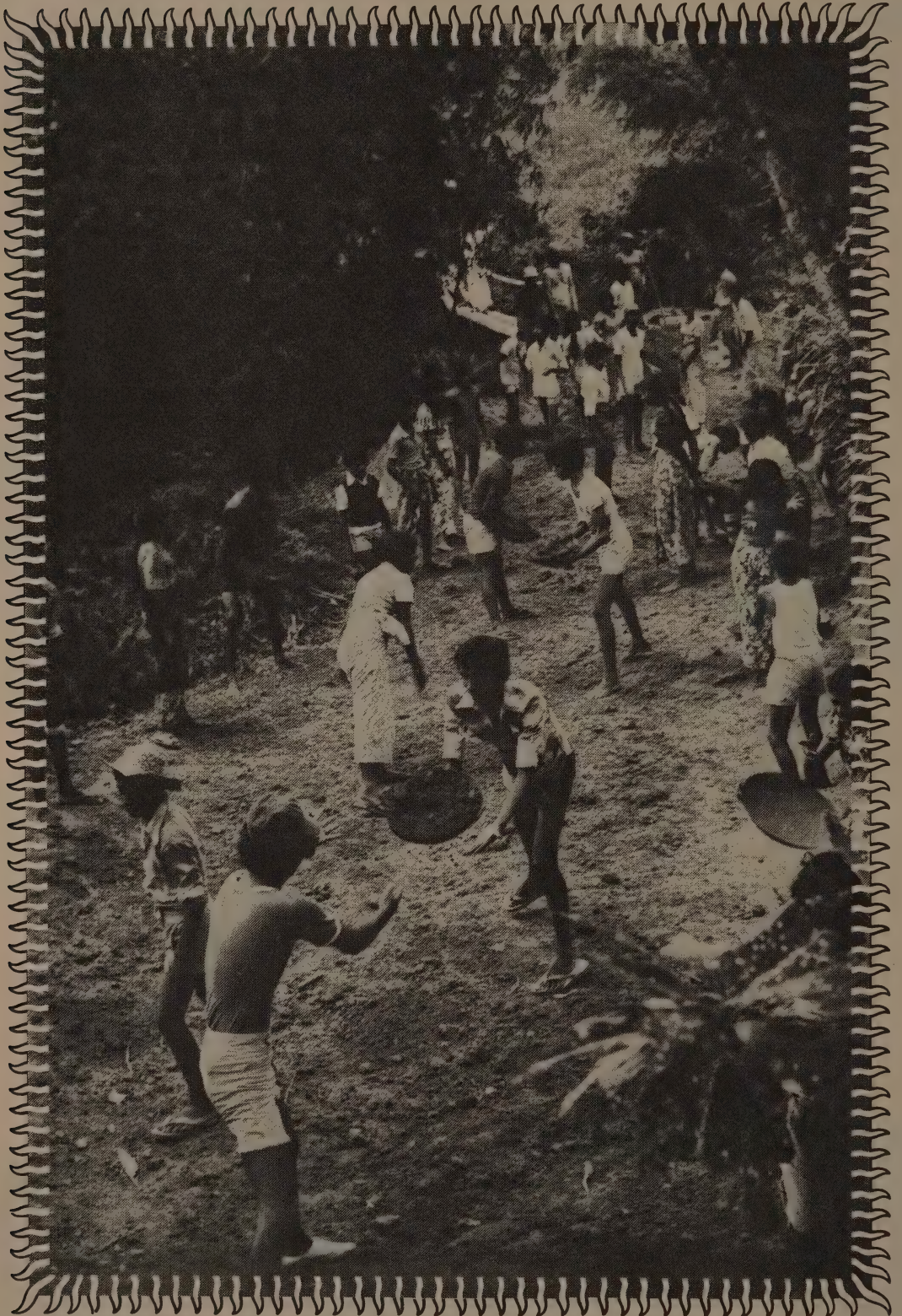
Earth moving, shramadana-style, to cut a jungle road.
